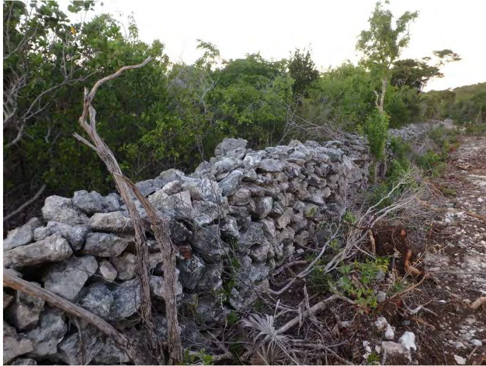
Old Rock Wall Abutting Unpaved Road
