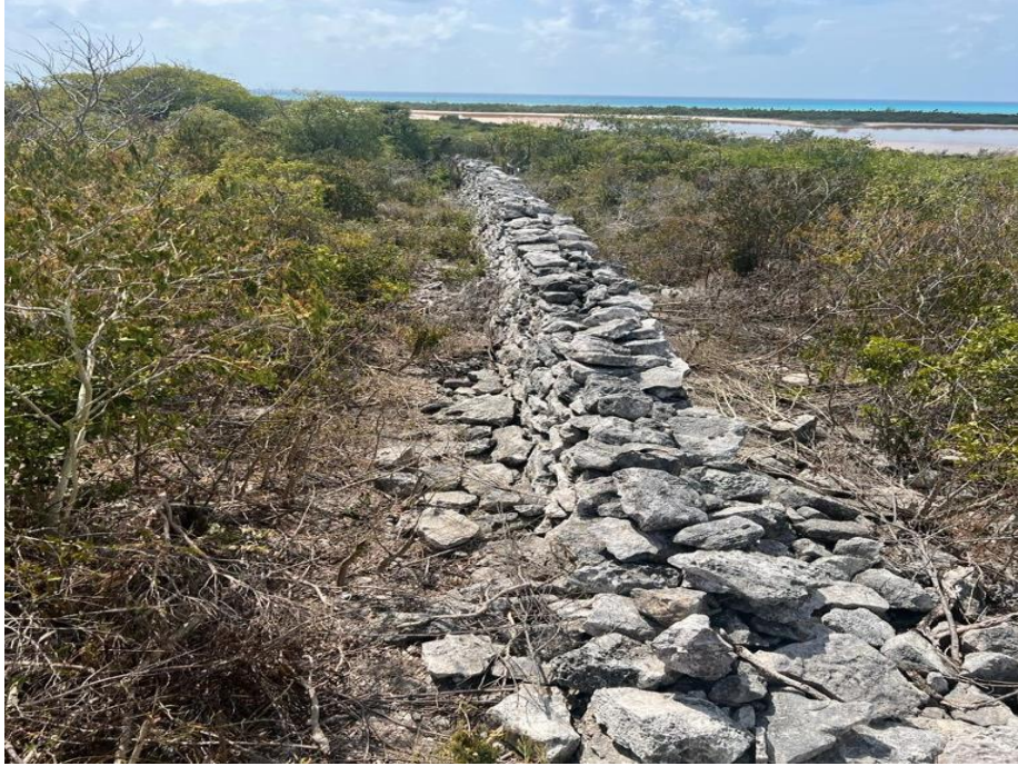
Figure 14: Boundary Wall in Palm Villa
