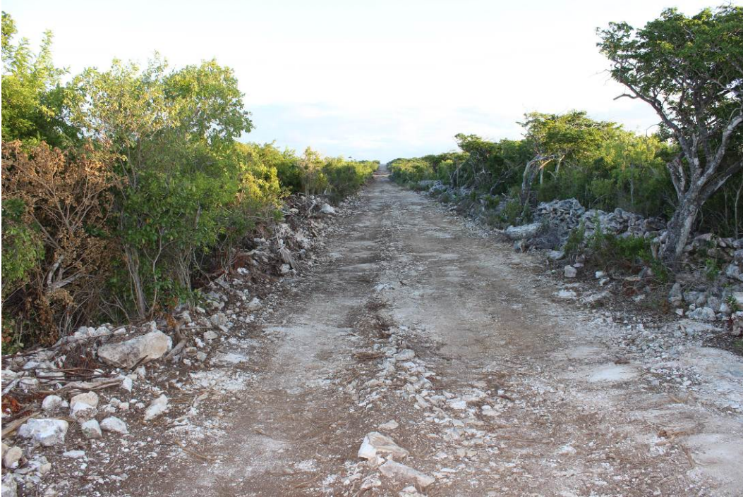
Photo 4-35. Typical Unpaved Road (December 9, 2022)
