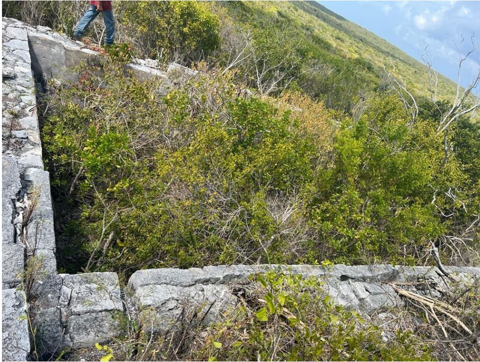
Figure 9: Building Structure in Palm Villa
