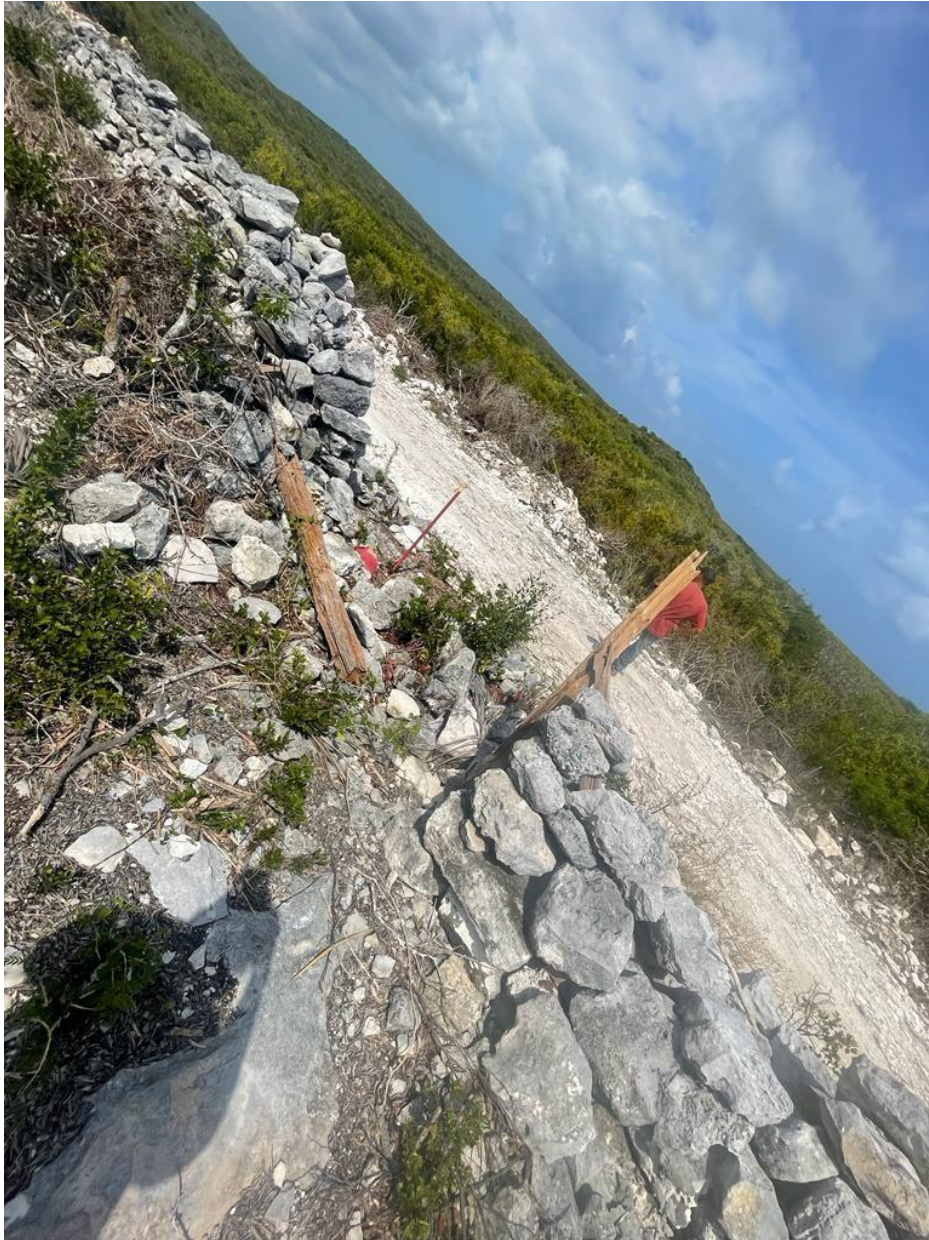
Figure 15 :: Boundary Wall in Palm Villa
