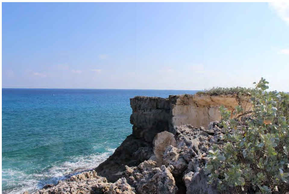
Steep Coastal Rock Bluff, Eroded, on Southeast Coastline
