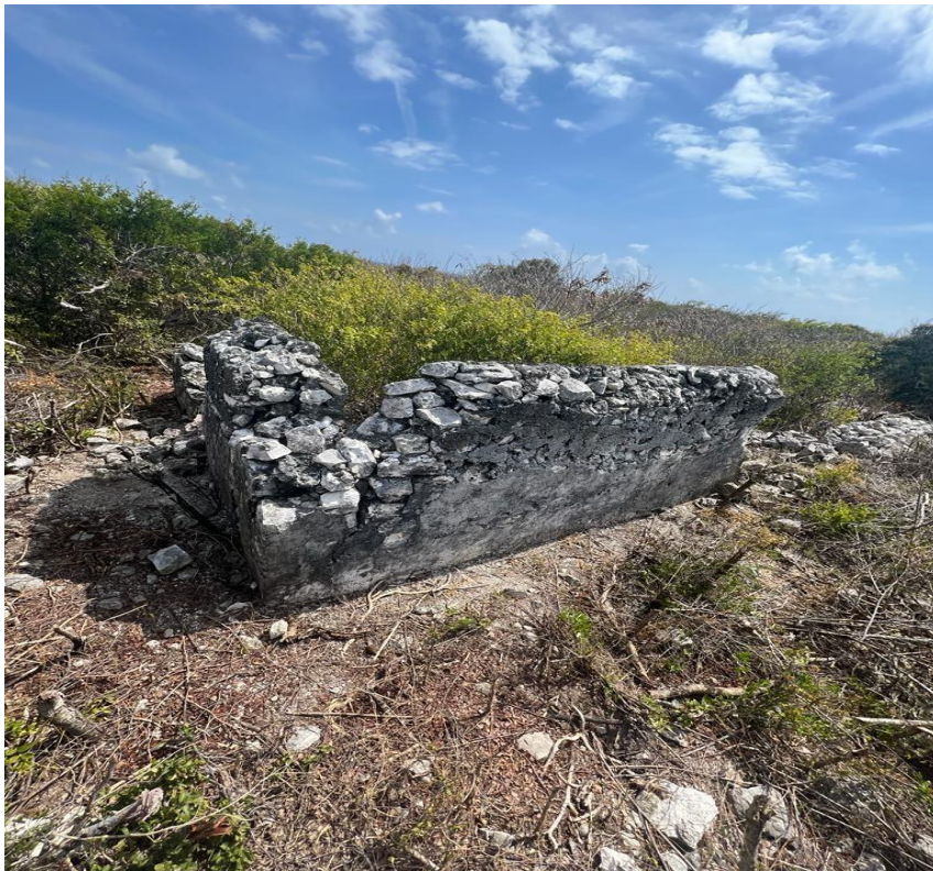
Figure 8: Building Structure in Palm Villa
