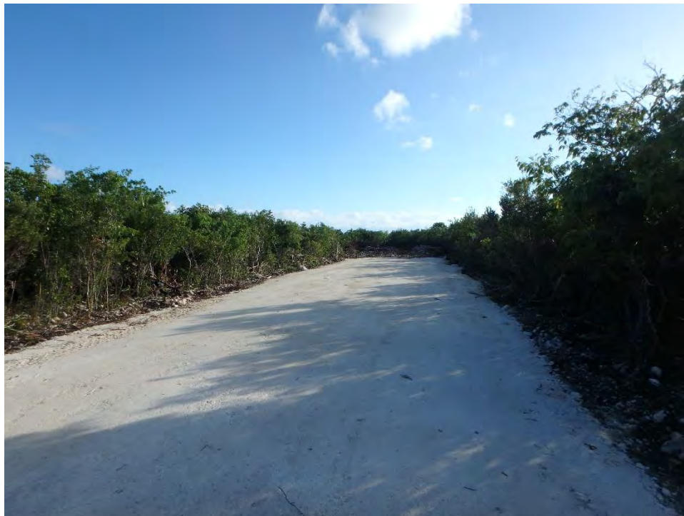
Former Landing Strip, Recently Resurfaced, View Looking East-Southeast
